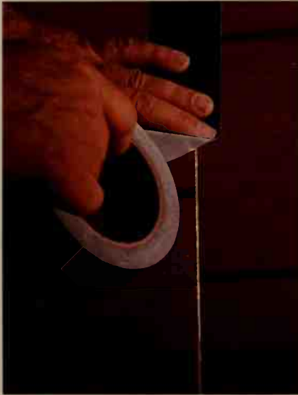
Dust is the enemy of good photographic quality. Limit the intrusion of dust by taping or caulking seams in paneling. Coat cement surfaces with a good sealer.
