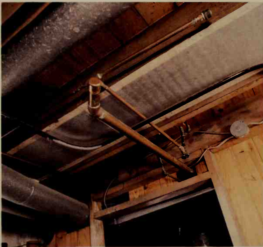
Overhead pipes are in the wrong place and cannot provide a drain.
