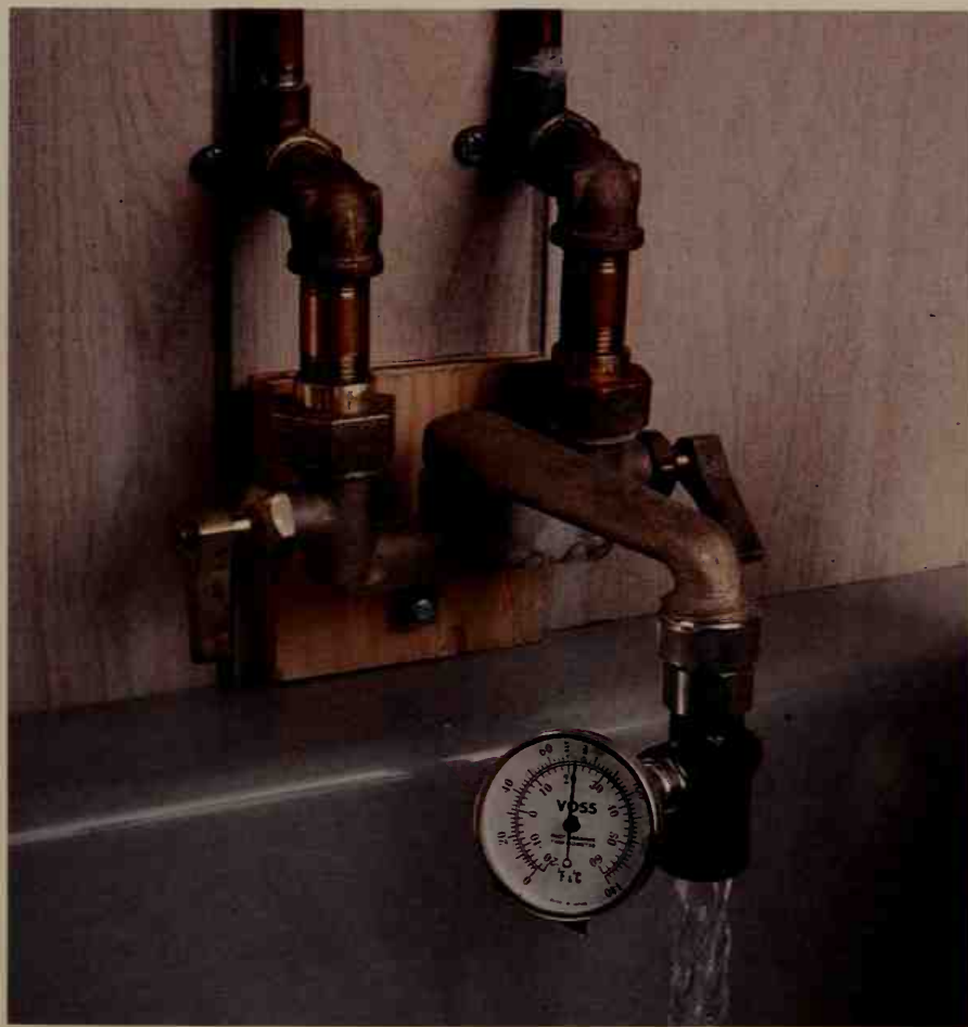
Our water faucet was converted from one intended to fit over a laundry tub. The text describes its conversion.
