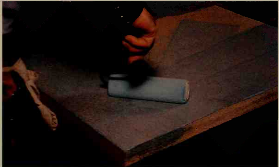
Preparing the top surface of the particle board with a sander is necessary to provide a better bond with the plastic laminate.
