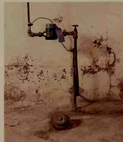
The clean-out cover will provide the drain opening that we need to serve our darkroom.
