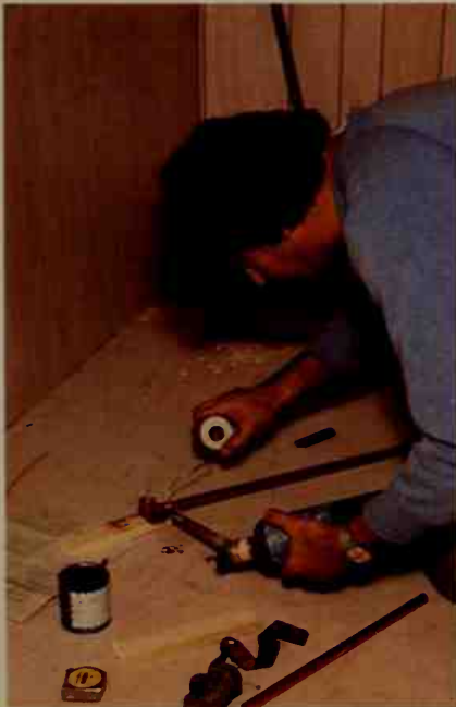
Our plumber is an expert at soldering copper pipe with roll solder and flux. If you prefer, you can use instant solder that comes in paste form with the flux mixed in. It's more expensive but it is easier to work with.
