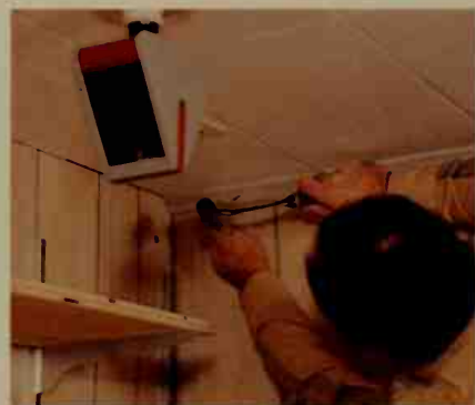
Mouldings cover the caulked seams.
