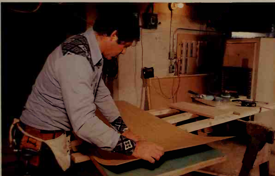
Our carpenter is an old hand at attaching the laminate to the particle board surface (see our comment on “slip sheets” in the text). Tapping with a hammer on a scrap of lumber disperses bubbles that might cause bumps in the finished top.
