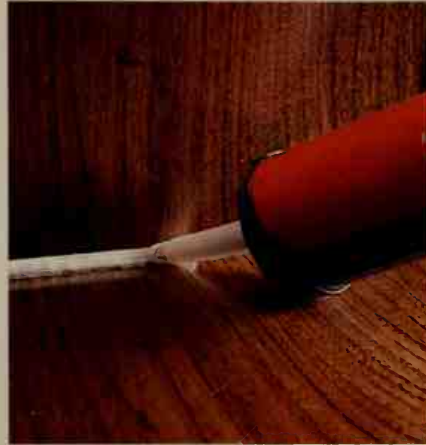
Dust is the enemy of good photographic quality. Limit the intrusion of dust by taping or caulking seams in paneling. Coat cement surfaces with a good sealer.
