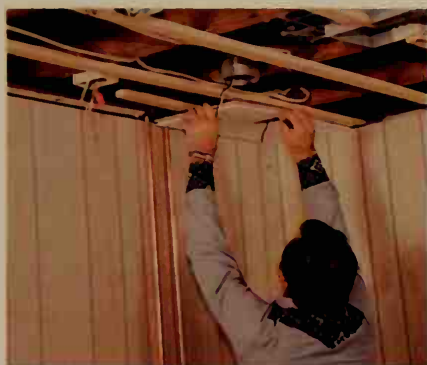
After completing the paneling, we proceed to install the ceiling tiles.
