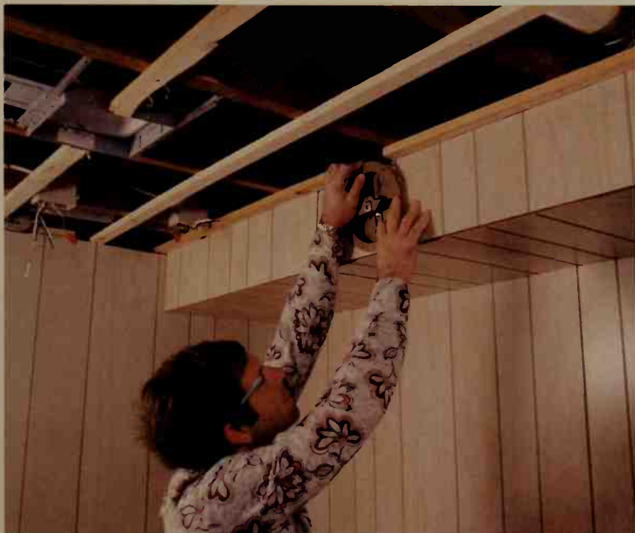
With the boxing in of the ducts completed, we refit the heat outlet and louvered finishing cap.
