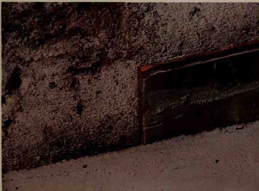
As the concrete sets up, we remove the temporary edging board to form a channel around the perimeter wall. When the concrete has cured as recommended, we will coat the floor with a sealer.
