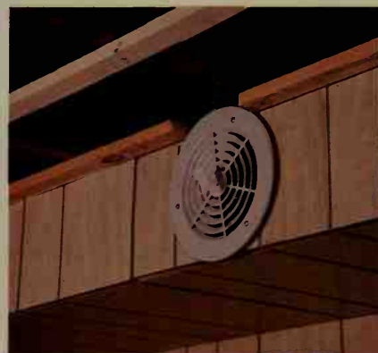
With the boxing in of the ducts completed, we refit the heat outlet and louvered finishing cap.
