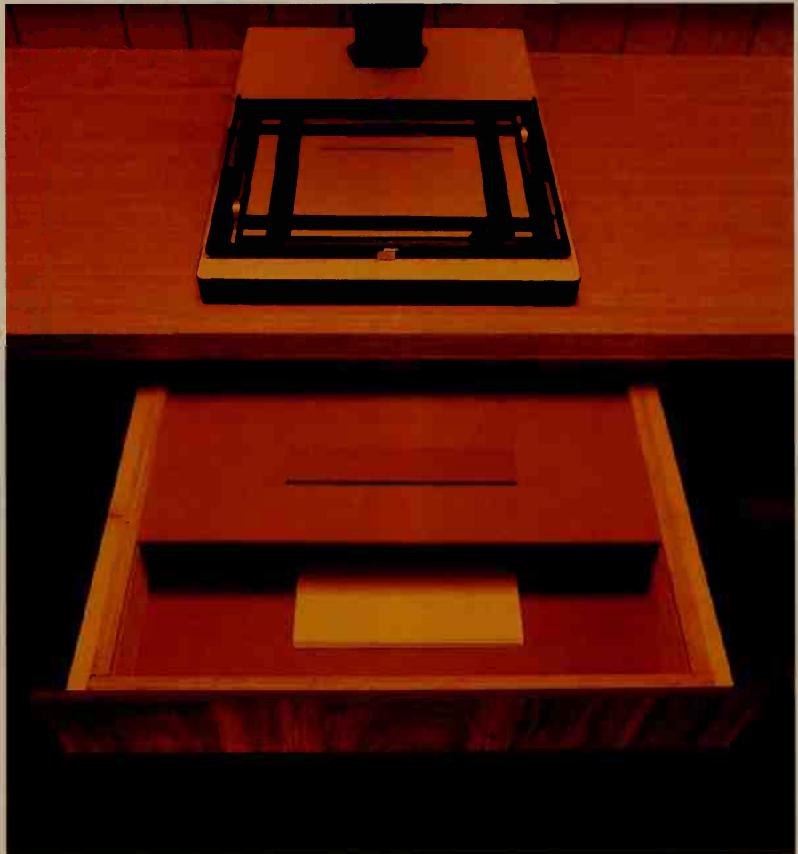
A completed dark drawer under the enlarger holds black-and-white paper ready for the easel. Note that we finished off our dark drawer with the false front that matched the other wood-grained doors and drawer fronts.
