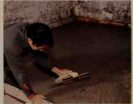
A straight 2 x 4 serves as a screed for evening the concrete surface. A steel tool provides the final finish.
