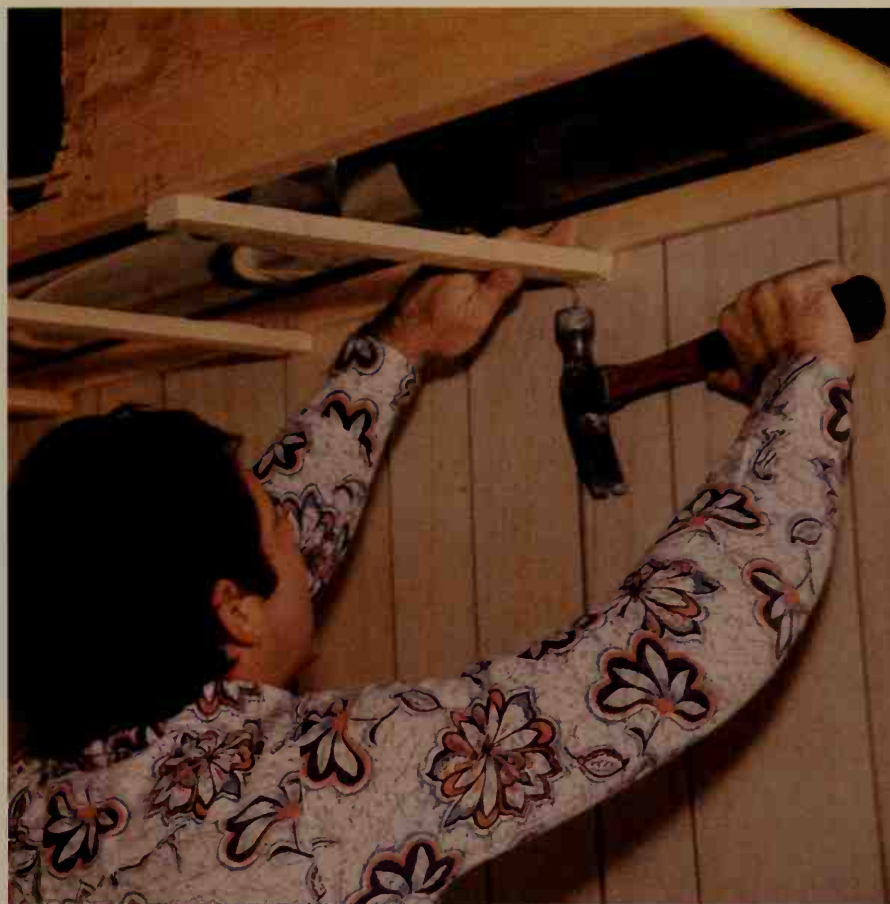
Boxing in the ducts proceeds with the use of filler strips as needed.
