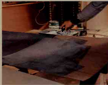
Our carpenter is an old hand at attaching the laminate to the particle board surface (see our comment on “slip sheets” in the text). Tapping with a hammer on a scrap of lumber disperses bubbles that might cause bumps in the finished top.
