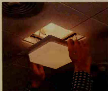
Fitting the opal diffusers over the lamps completes the ceiling installation.
