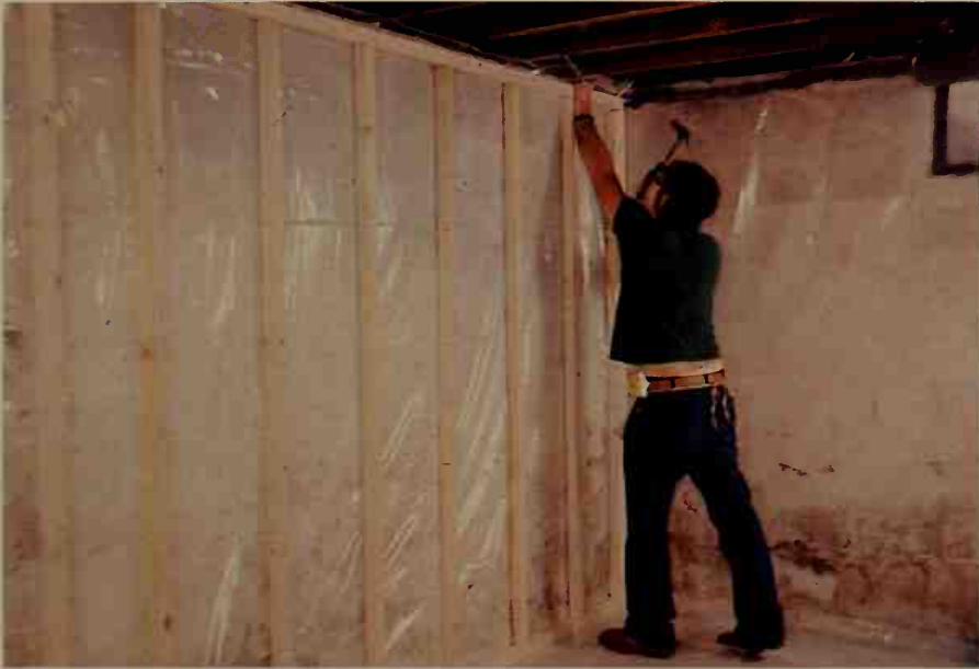
Final step in erecting the 2 x 2 framing is to make it plumb (using shims to space it from the wall as needed) and to nail it into place. Each of the three exterior walls gets this treatment.
