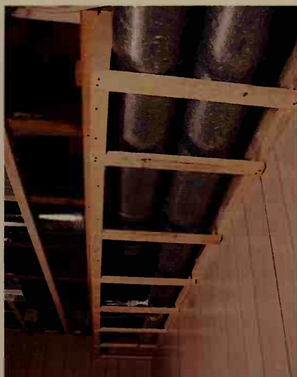
Boxing in the ducts proceeds with the use of filler strips as needed.
