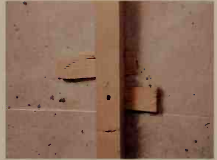
Final step in erecting the 2 x 2 framing is to make it plumb (using shims to space it from the wall as needed) and to nail it into place. Each of the three exterior walls gets this treatment.
